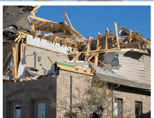
Brick homes suffered mild to devastating damage.
